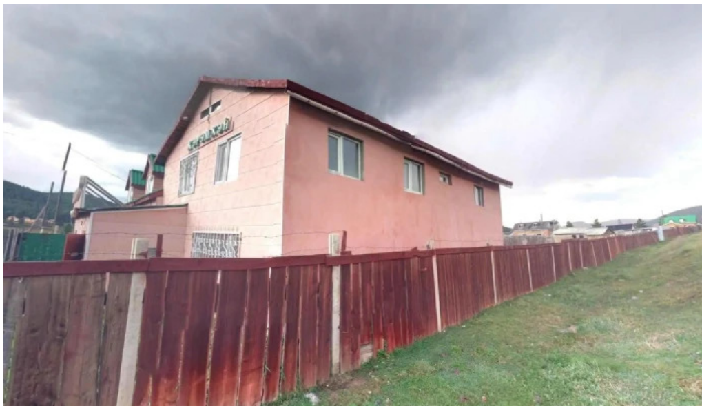
Baga bayan complex gudamzh kharakh bolon 360deg
